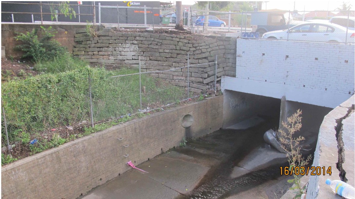
Figure 3.2 Duck Creek Channel & Culverts under intersection of William Street & Blaxcell Street
