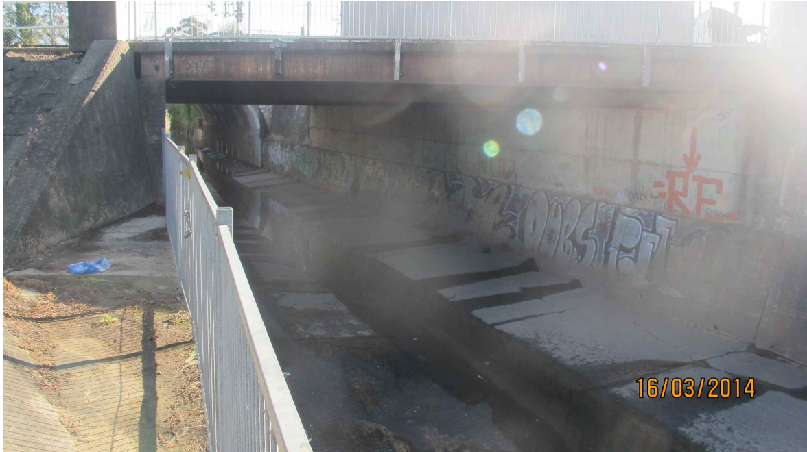
Figure 3.6 Duck Creek Culverts Under Memorial Park Drive & Main Western Railway Line
